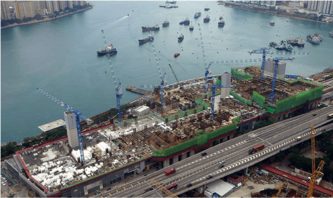
Ocean Pride construction progress in January 2016 (four months after work commencement)
