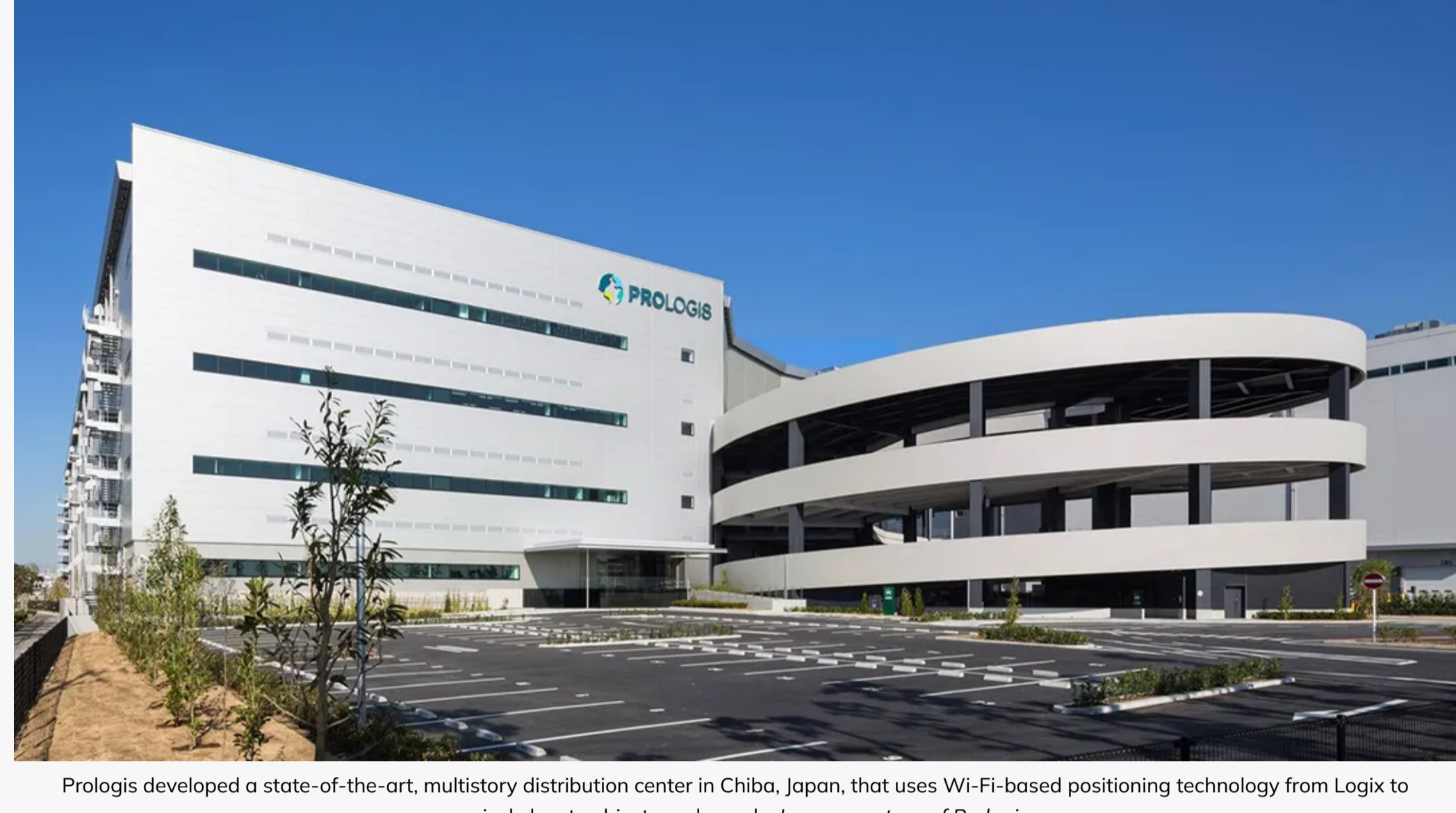
Prologis developed a state-of-the-art, multistory distribution center in Chiba, Japan, that uses Wi-Fi-based positioning technology from Logix to precisely locate objects and people. Image courtesy of Prologis
